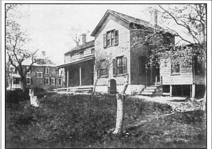
The Martin Quackenbush homestead, 184 Myrtle Avenue, in a photograph taken about 1907-1910.
