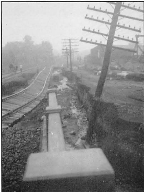
Looking west from top of West Crescent Avenue overpass.
