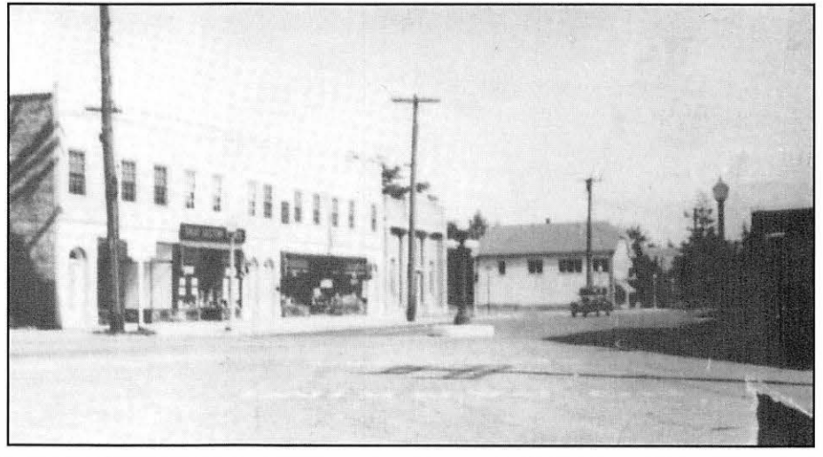
Below, the same view on September 26, 1932 after the original Winter Building had been moved to High Street, and the new Winter Building was erected on the site.
