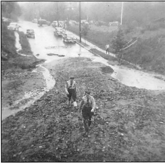
Looking north from railroad tracks on top of the West Crescent Avenue Erie underpass at State troopers investigating flood damage.
