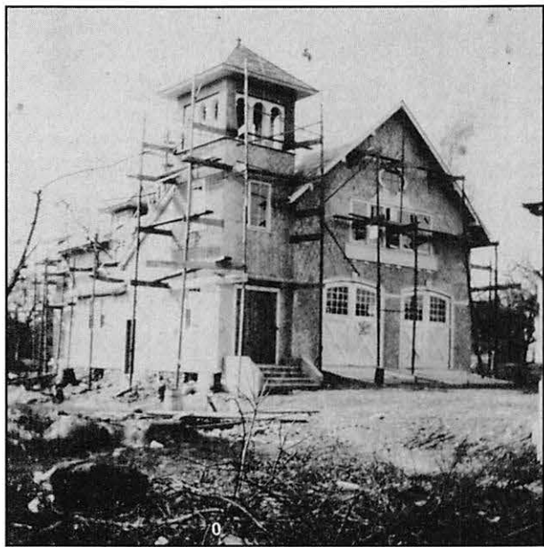
The Allendale Fire House under construction in 1913.
