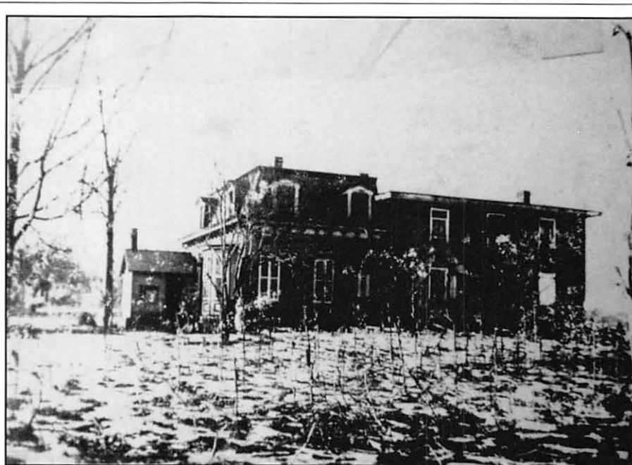
The Elias Doolittle house about 1885. The house, which may have formerly been a hotel, stood near the site of today's Railroad Station.
