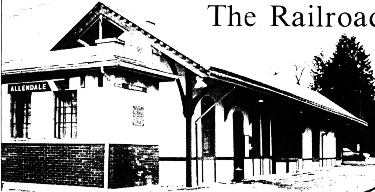
The present railroad station is actually the Borough's third depot. Two previous buildings were located on the northwest side of the tracks.
