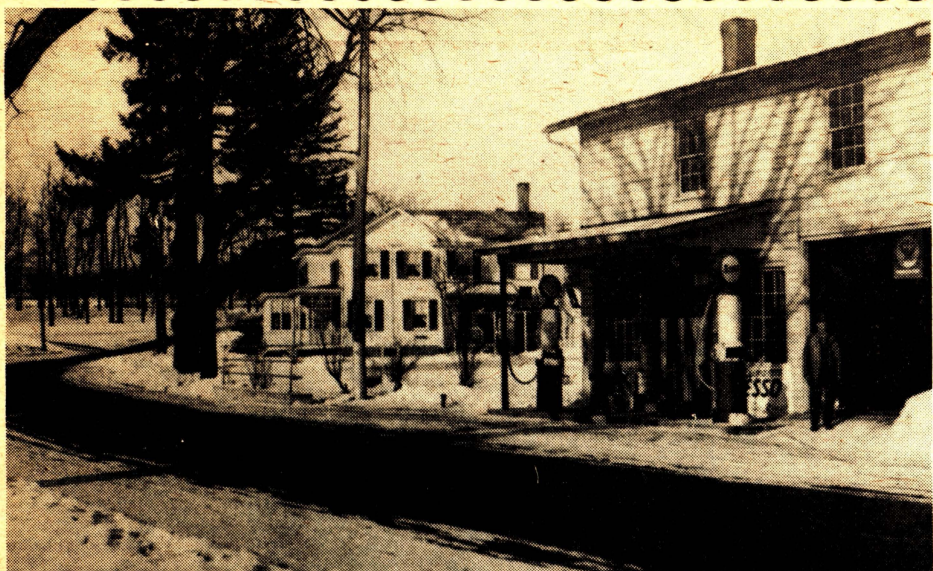
Milton Packer stands by the gas pumps in 1935 and proudly shows visitors what remains of the old foundry and mill equipment from Packers. (Today the building houses Joseph Murphy Real Estate and Petit Point Junction.) At left is the Will Packer home, now the Coach House.
